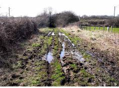
Figure 3.3. Trail divergence. User avoidance of muddy conditions lead to trail divergence and a wider track. *Source*: Oliver Dixon via Wikimedia Commons.
