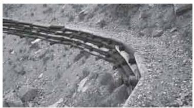
Figure 4.3. Crib wall. Crib walls are retaining structures used in trail construction to create level trails across sloping terrain. *Source*: United States Department of Agriculture, Forest Service, Technology and Development Program, Trail Construction and Maintenance Notebook, Woody Hesselbarth, Brian Vachowski, and Mary Ann Davies. No. 0723-2806-MTDC (2007), http://www.fs.fed. us/t-d/pubs/htmlpubs/htm07232806/page12.htm (accessed April 3, 2014).
