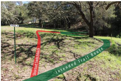
Figure 3.2. A shortcut switchback. This is common without proper barriers installed. *Source*: Author.
