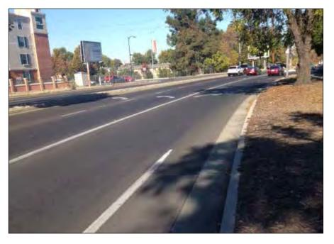
**Figure 3.22**: Senter Road Bike Lane Ends Abruptly Before Reaching Keyes Street.
