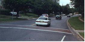
**Raised Crosswalks** are flat areas raised to the level of the sidewalk with ramps along the sides.
