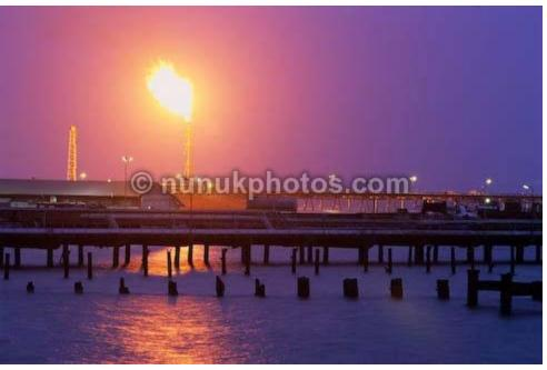
Refineries and chemical plants are equipped with these to burn off waste, especially during accidents. In this case, the accidental release gasses are routed to flare to be burned off.
