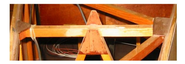
Figure 3: Reinforced Truss Joints (Nordin, 2006)
